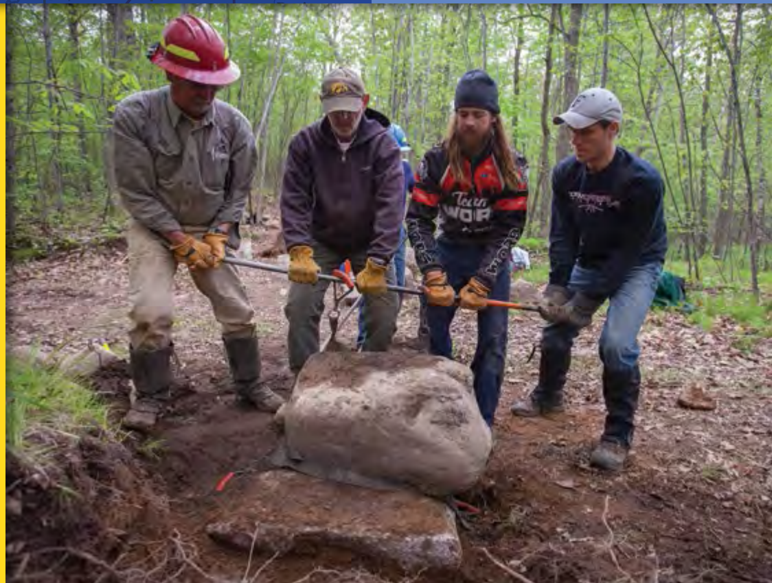
One of the many rocks appraised for its usefulness is carefully slid into place by volunteers. A hand-crafted, rock staircase, like this one, requires teamwork and well-established safety protocols. Photo by Cameron Gillie.
