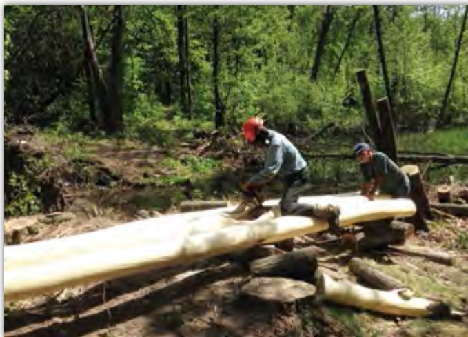
A chainsaw certified volunteer adeptly shapes timber to be used for constructing a bridge. Photo by Michael Maziarka.
