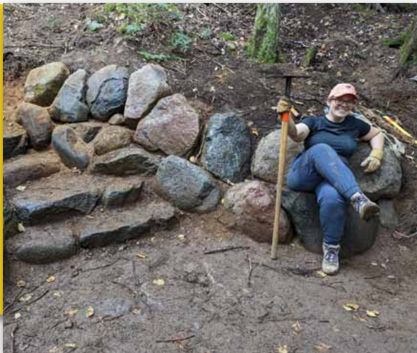
A volunteer shows off the new stone staircase and retaining wall. Photo by Dave Caliebe.
